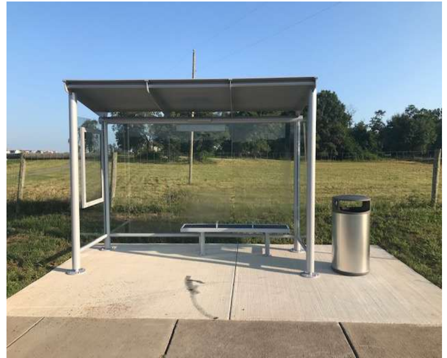
Bus shelter by the BSA leased area.
